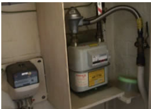
Asbestos panelling around a gas meter
