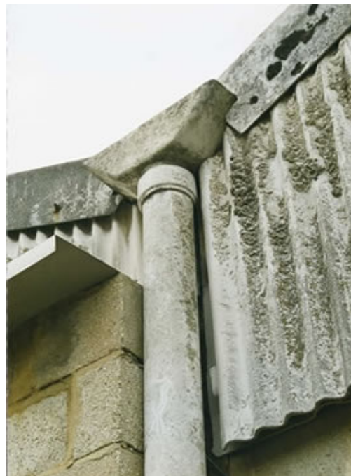
Asbestos cement downpipe, hopper and profile sheet
